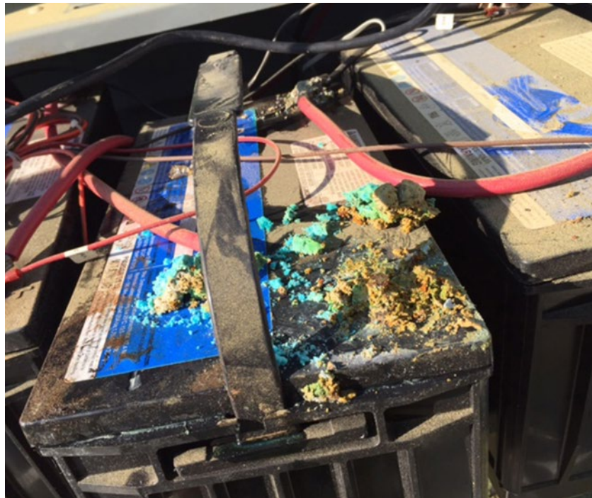
Figure 14 – Battery Corrosion
